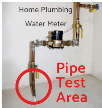
Your water meter could be located inside your home's basement or crawlspace. The service line will enter the house from underground through the floor or foundation wall, before connecting to the water meter. There will be shutoff valves on one or both sides of the water meter. Residential service lines are ¾ to 2 inches in diameter.
